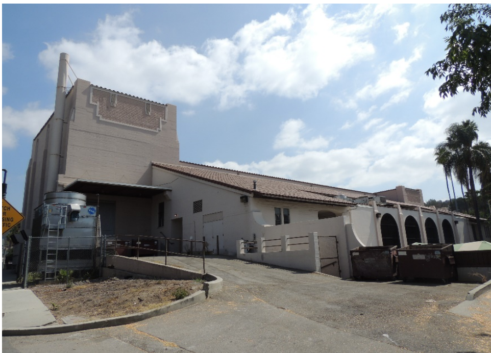
Figure 15. Exterior, west and south façades, view looking northeast. September 2016, TGHS.
