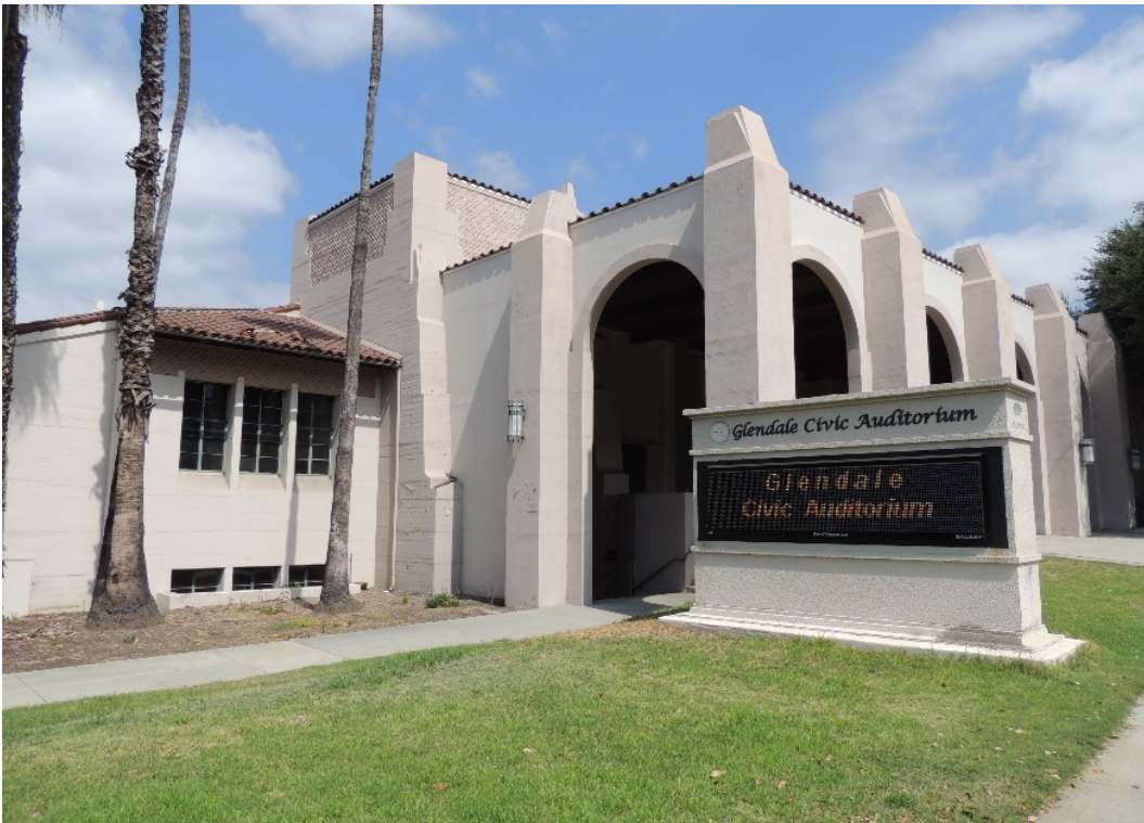
Figure 10. Glendale Civic Auditorium, exterior, east arcade, view looking northwest. September 2016, TGHS
