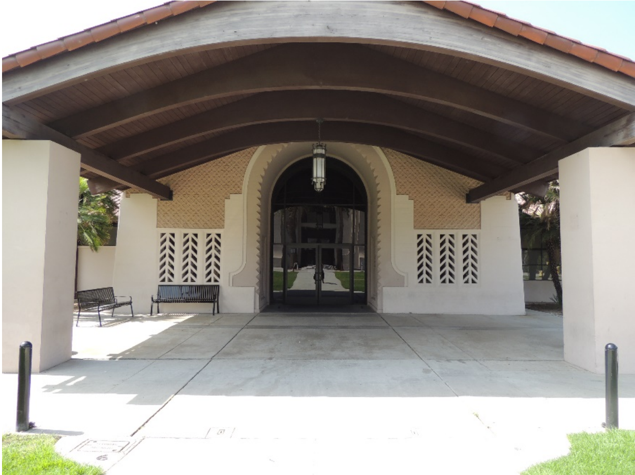
Figure 12. Glendale Civic Auditorium, exterior, north façade, primary entrance, view looking south. Detail of concrete grilles and Moorish cast geometric patterns. View of same main entrance as Figure 12 before removal of 1963 entrance loggia. Note delicate texture of concrete on upper portion of wall prior to 2017 paint scheme. September 2016, TGHS.
