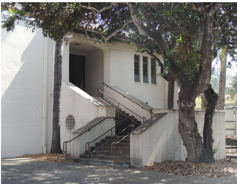
Figure 16. Exterior, south façade, east exterior stair, view looking northeast. Note the segmentally arched, recessed doorway. September 2016, TGHS.
