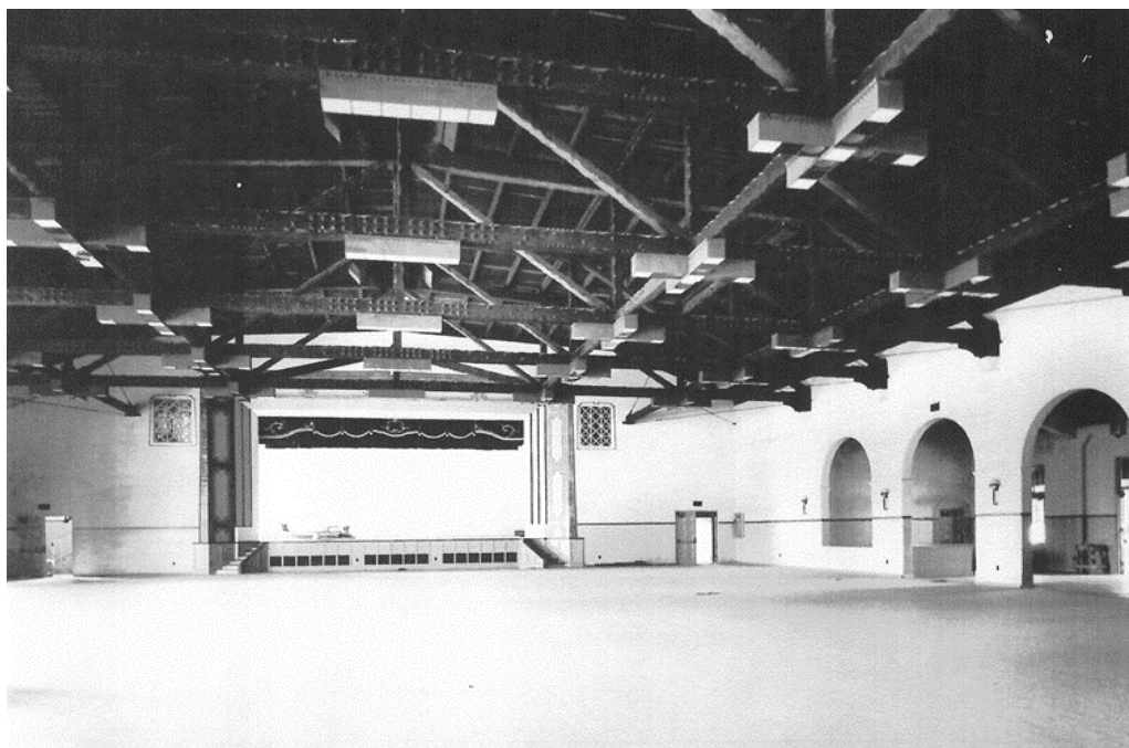
Figure 7 Verdugo Municipal Recreation Center, interior detail, view west, c. 1938. Source: Lisa Grundfor.
