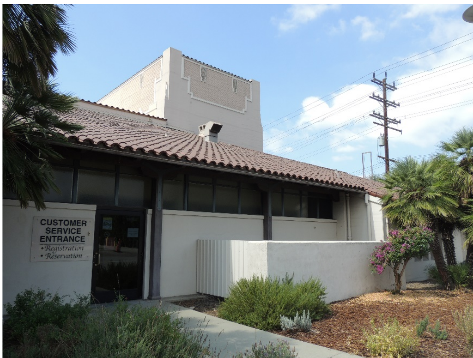
Figure 13. Exterior, north façade, enclosed west corredor , view looking southwest. September 2016, TGHS.
