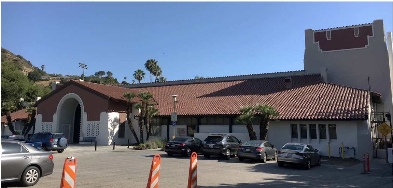
Figure 2A: Verdugo Municipal Recreation Center, north façade, view southeast. Entrance loggia added in 1963 had been removed, revealing original entrance bay. May 2017, TGHS.
